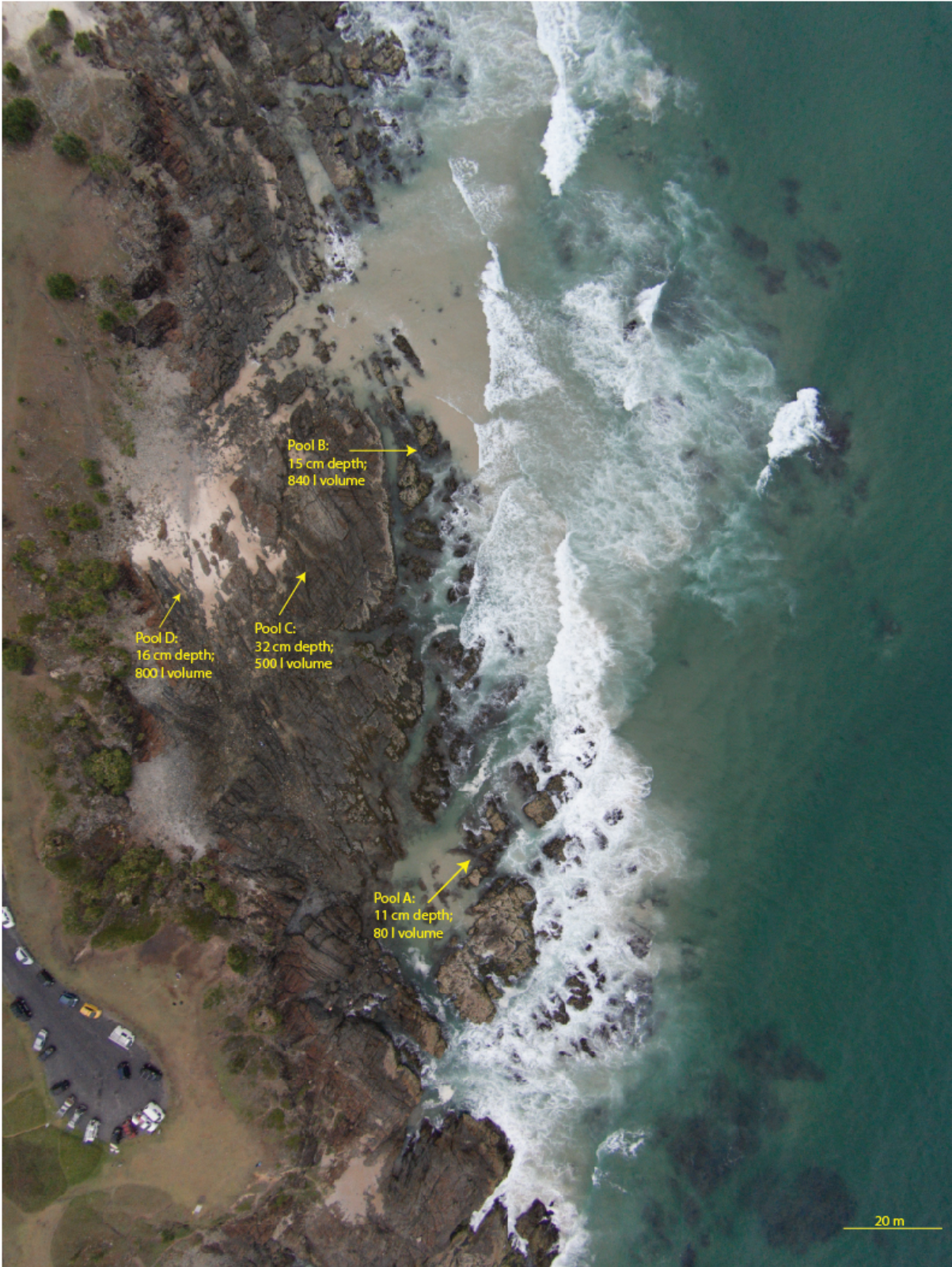
Supplemental Figure 1: Aerial view of the tidal platform and sampling pools at Hastings Point, NSW.
