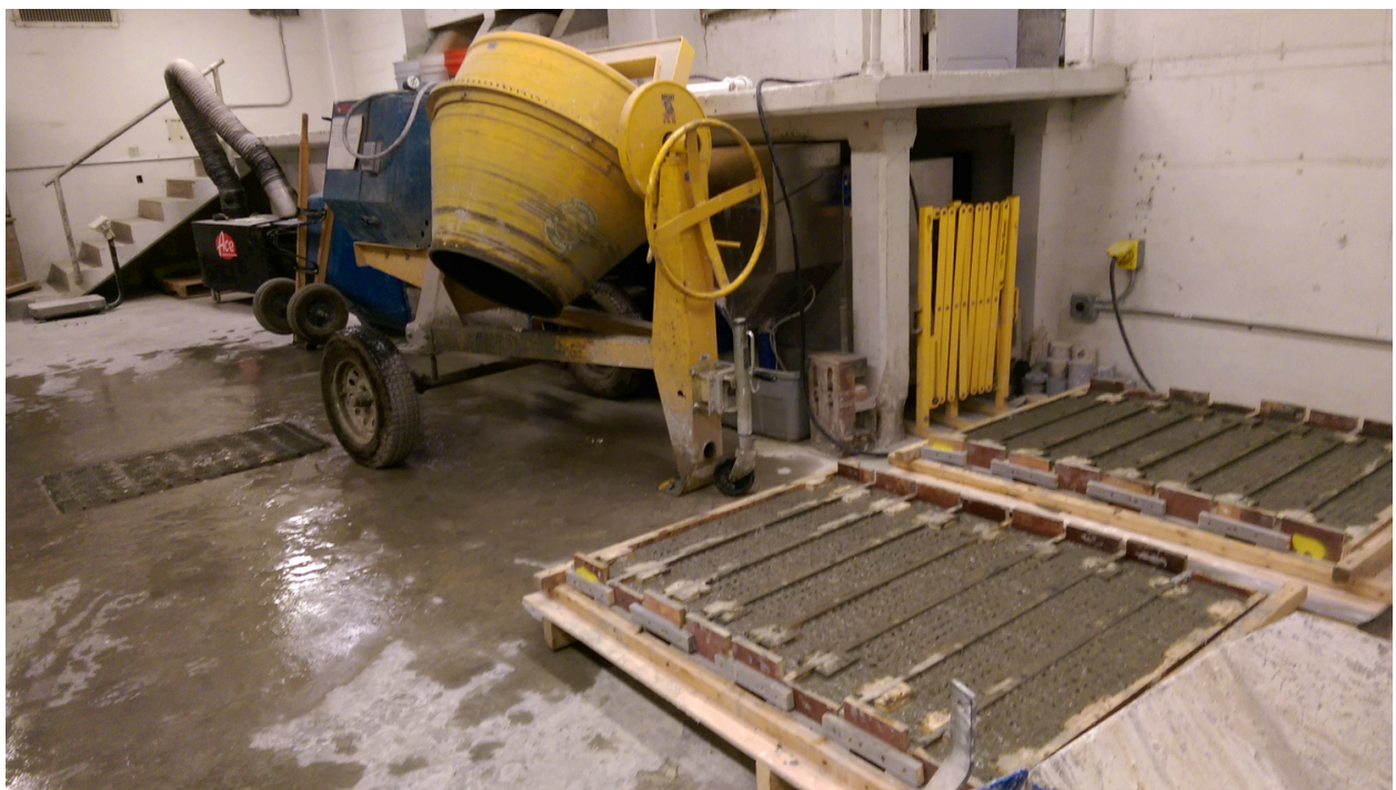
Figure S10. Poured concrete.
