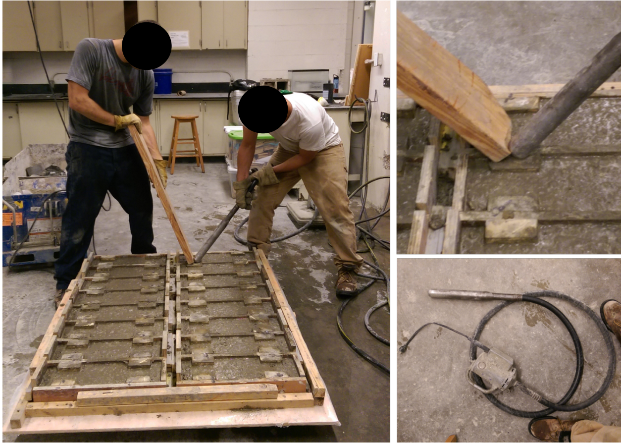
Figure S9. After pouring, apply the vibrator to eliminate bubbles. A piece of scrap can be used to keep the vibrator from sliding into the concrete.
