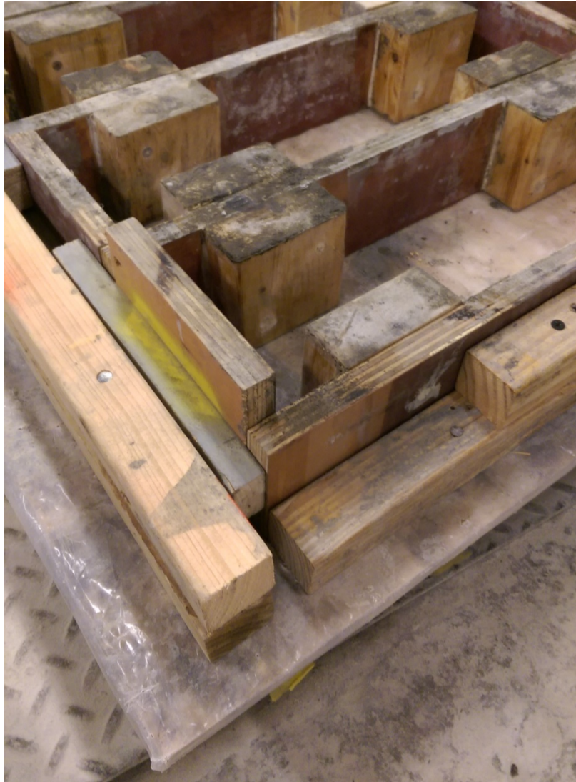
Figure S7. The corner of a small mold unit ready for pouring. Note the yellow paint indicating the orientation of the end side plate.
