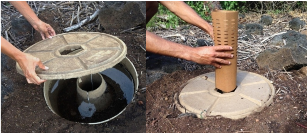
Figures 27 & 28. Lid and protector being placed for protection
